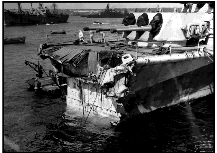
USS Pittsburgh (CA 72) shown missing bow in Guam, next to USS Duluth (CL 87). Damaged during the 5 June 1945 typhoon
