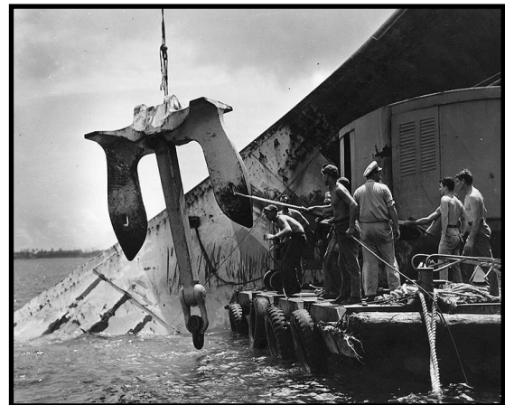
Lifting the starboard anchor from the cruiser's detached and capsized bow, during salvage operations at Guam, circa June 1945
