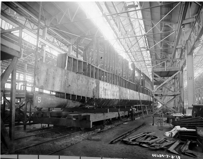
Eagle Boat under construction at the Ford plant
