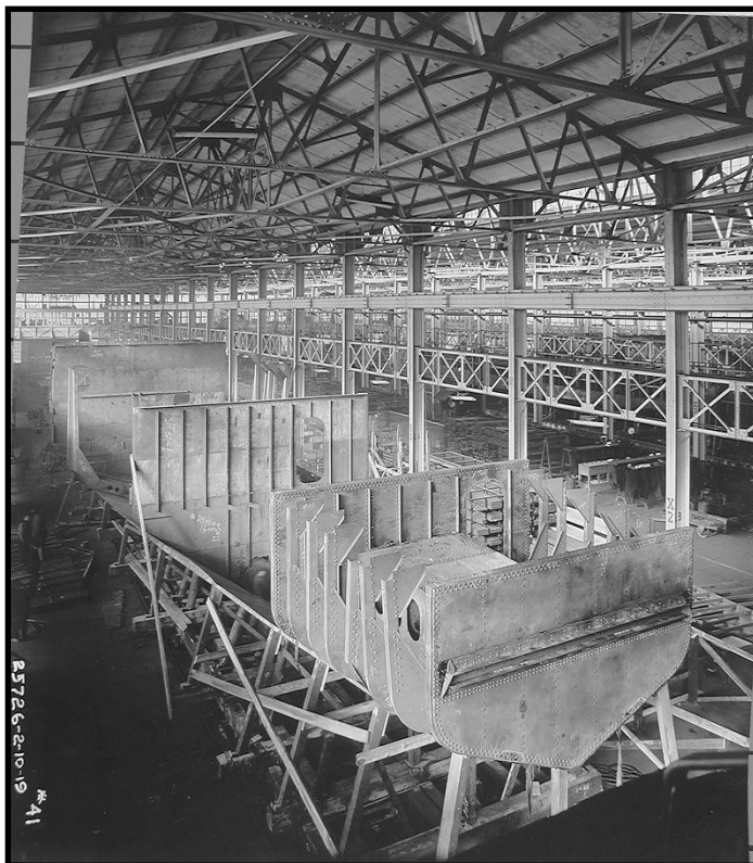
Eagle Boat under construction at the Ford plant
