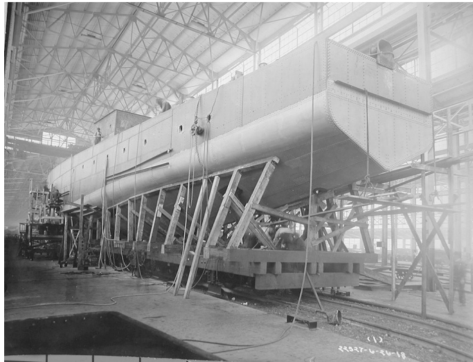
Eagle No. 1 under construction , 16 June 1918
