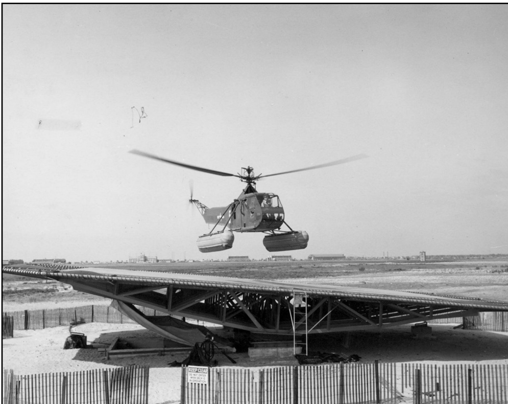
USCGC HNS-1 Hoverfly during trials on a rocking platform
