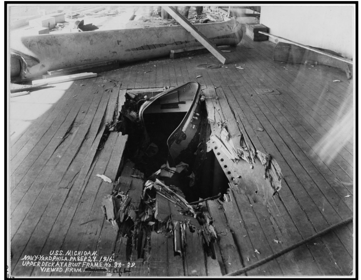
Deck Damage Following Gun Explosion
