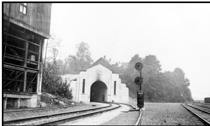
CPR Dunsmuir tunnel west portal
