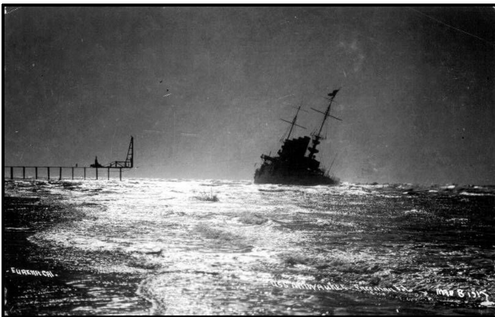
Postcard of USS Milwaukee stranded on Samoa Beach, 8 MAR 1917. Note the pier being built to facilitate salvage of the Milwaukee .
