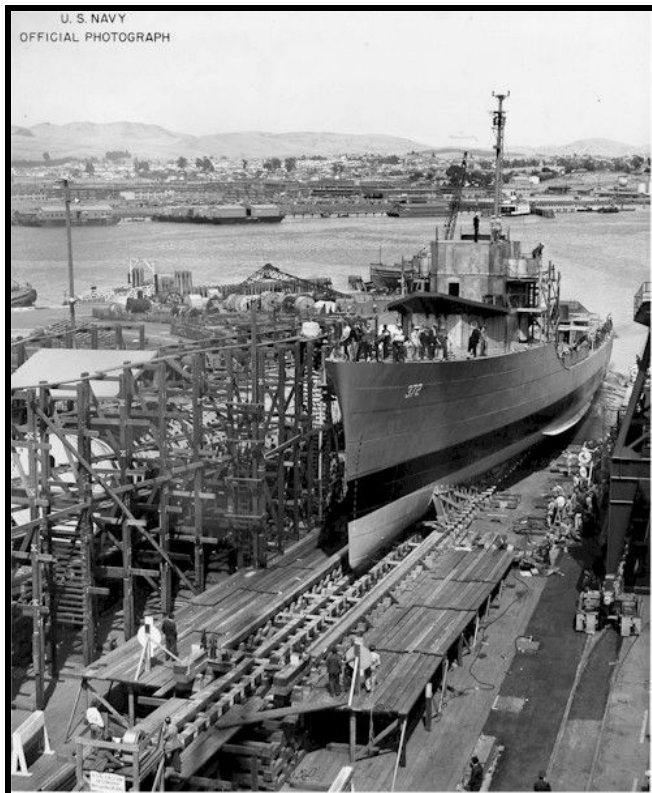
The USS Cassin (DD 372) is half way down the building was at Mare Island Navy Yard on 16 June 1943. The partially completed hull of the USS Spadefish (SS 411) is to the left behind the staging.
